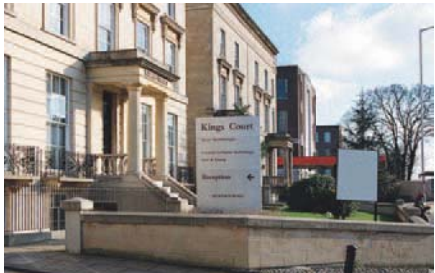
Wipro Development Center at Reading, UK
